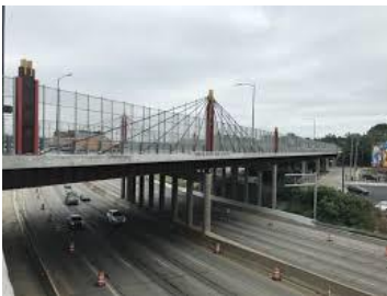
Martin Luther King Bridge
